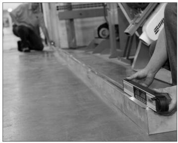
Align the "PAL" Tool with Windscreen Base Shoe and point toward the Laser Target set at opposite end.
